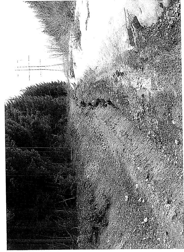
Damage to Easton Ridge Road from Runoff - April 05
