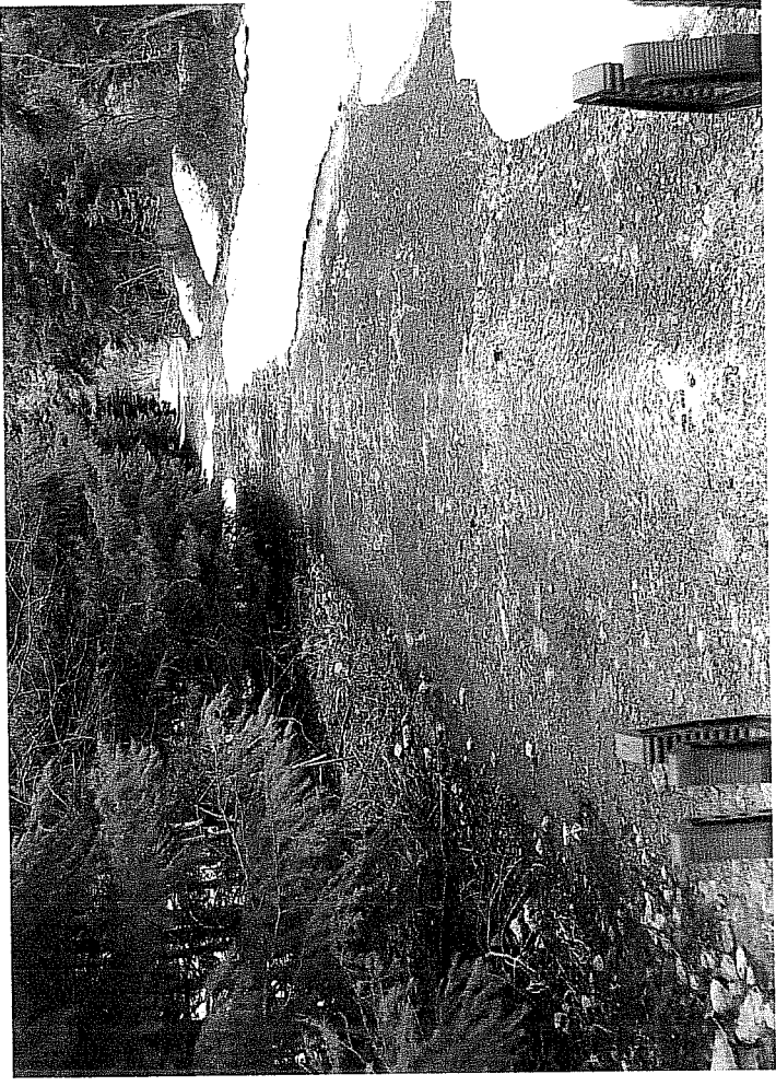
Damage to Easton Ridge Road from Runoff - April 05
